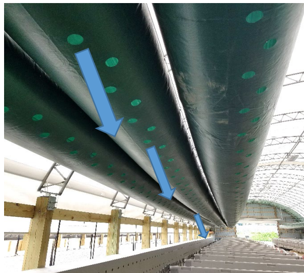
Figure 1. Polyethylene ventilation tubes in a greenhouse calf barn introduce air in mild and hot seasons. Blue arrows represent air streams introduced by the tube fan ventilation system.
